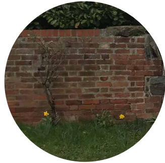
Red brick wall boundary
