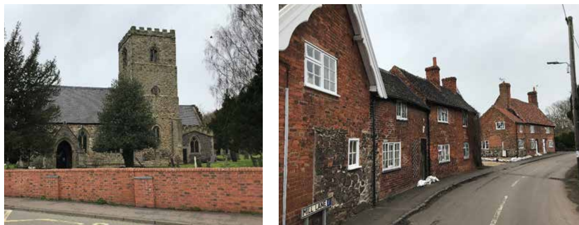
Figure 12: Long Whatton Conservation Area example buildings
