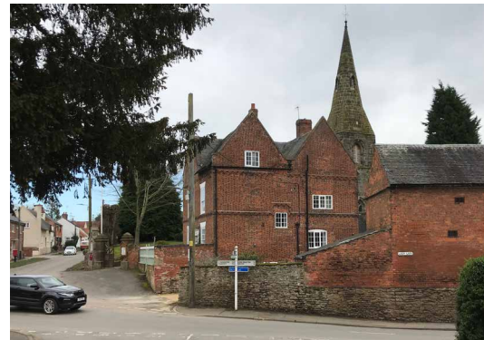
Figure 8: Grade II listed Cross Farmhouse and grade II* St Michaels Church
