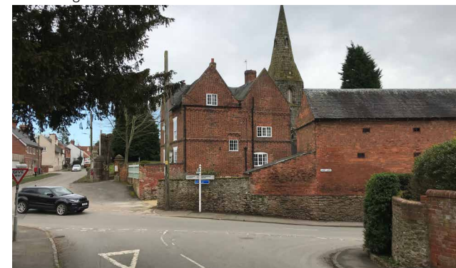
Figure 18: Example of a tertiary route, footpath on both sides but no hedgerows
